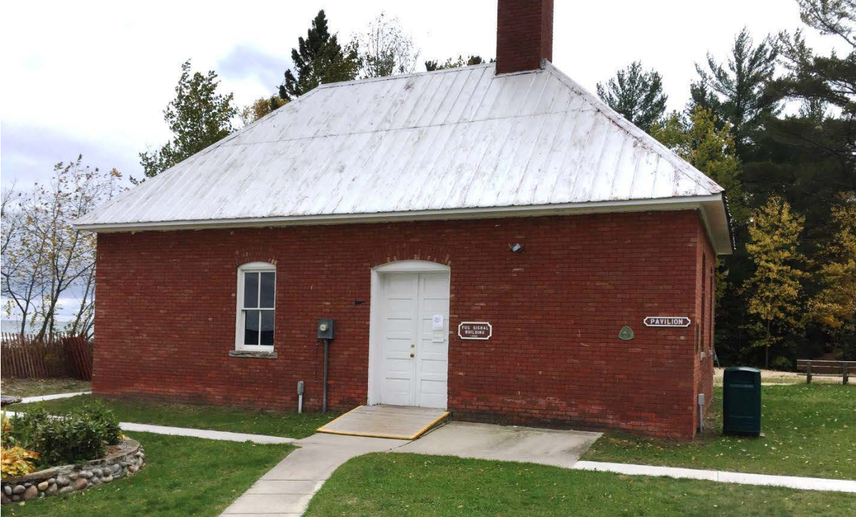
Former Fog Signal Building, converted into a Pavilion. LWCF plaque is on the right side of the building.
