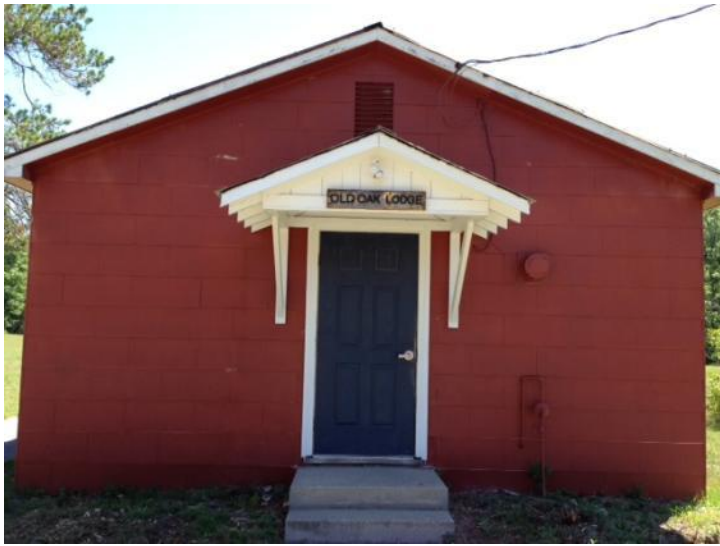
Entry (West Elevation)
