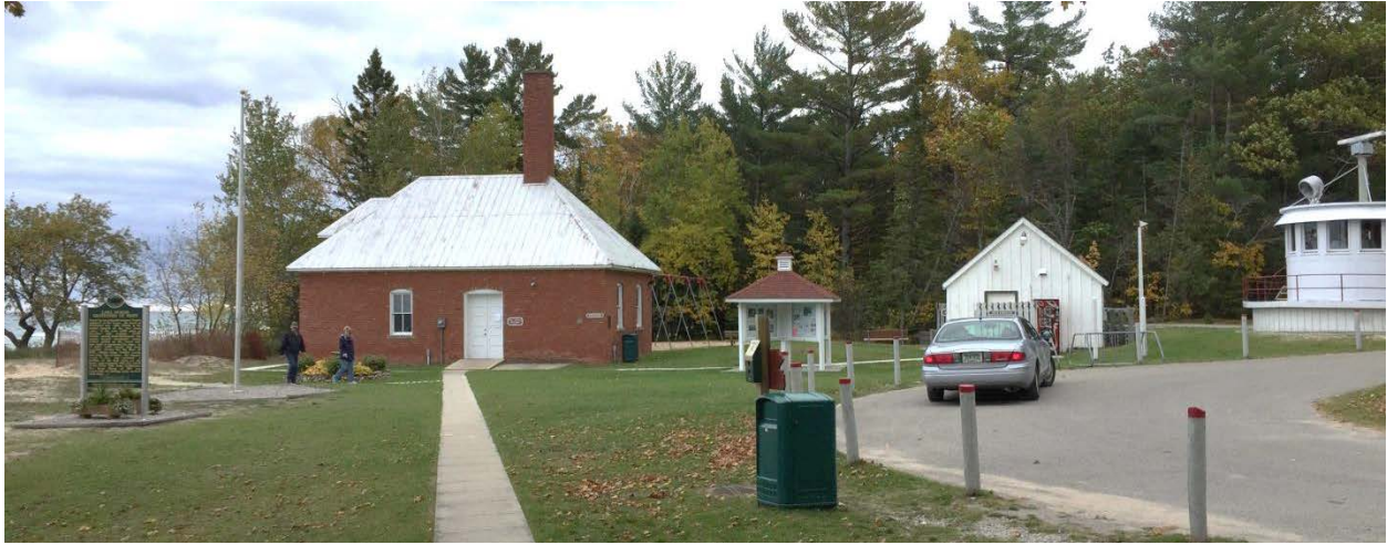
Looking south at the former fog signal building, pavilion, and restrooms/changing rooms
