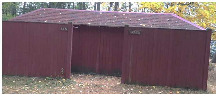
Restrooms near the open pavilion.
