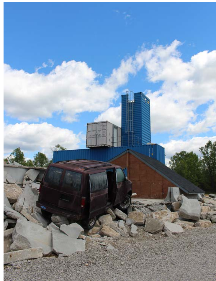
The Combined Arms Collective Training Facility (CACTF) at Camp Grayling JMTC consists of numerous structures to train soldiers in Urban Operations capabilities.
