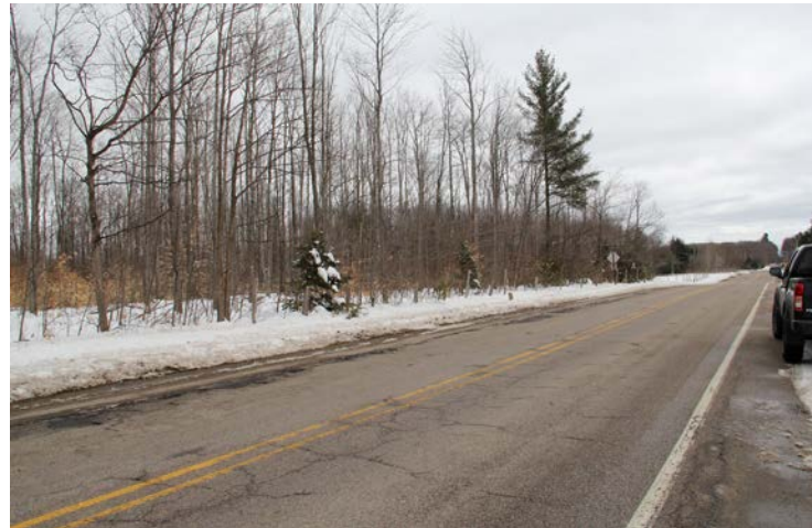
Harsh winters and the spring freeze/thaw cycle cause wear and tear on local roadways.
