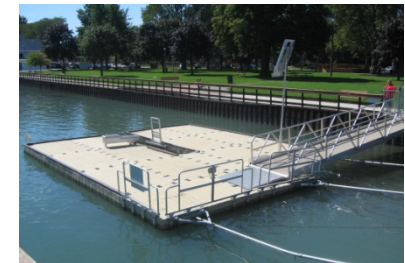
Water Trail ADA Accessibility Guidelines: Whenever possible, local water trail planning initiatives should include ADA-accessible kayak launches. Simple launches like the one pictured above in Wyandotte, Michigan, can be purchased for around $30,000.
