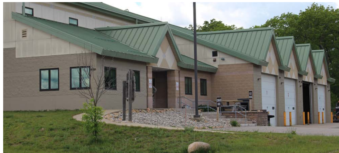
Alpena CRTC has an operations building on Camp Grayling JMTC.
