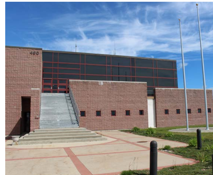
Base operations building.
