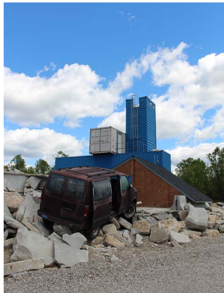
The Combined Arms Collective Training Facility (CACTF) at Camp Grayling JMTC consists of numerous structures to train soldiers in Urban Operations capabilities.
