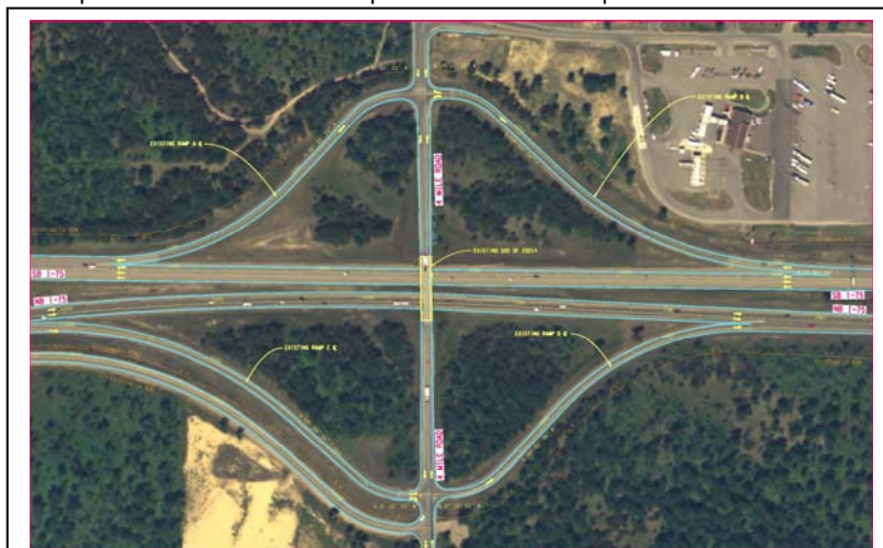
Figure 5-9: Existing I-75 & 4 Mile Road Interchange
