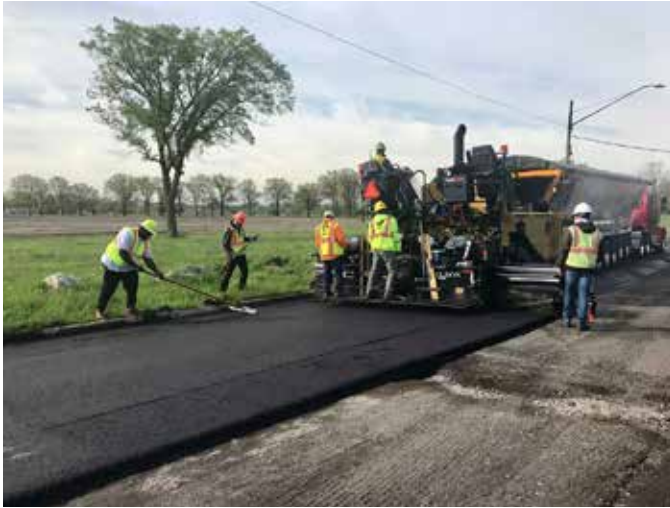
Repaving roadways can make less used roads more comfortable for users.
