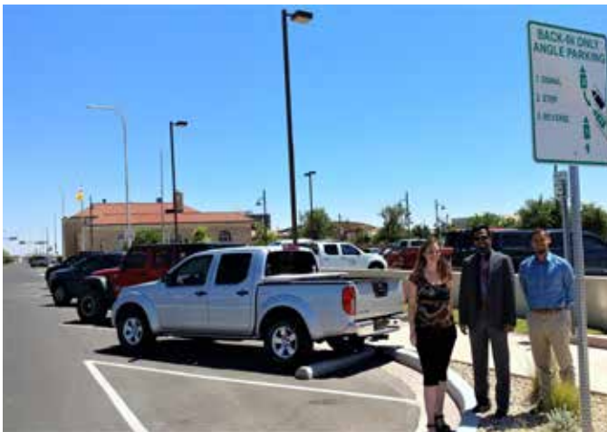
On-street parking improvements, such as reverse angled parking, can improve safety in busy commercial areas.
