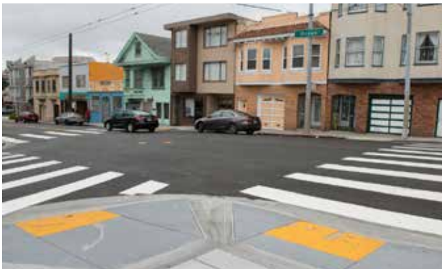
High visibility crosswalks can notify motorists of the potential for pedestrian crossings.
