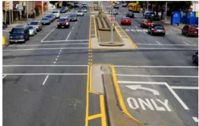
Medians and dedicated left turn lanes can help reduce crashes and improve the efficiency of a street.
