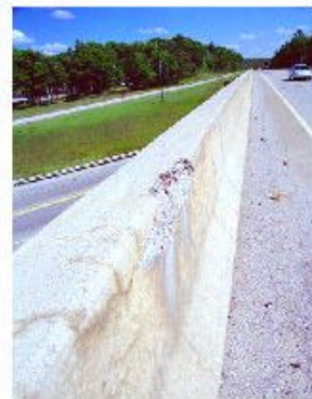
Figure 5.8. Illustration of a tube-style see-through guardrail (l), and a photo of a concrete bridge barrier in need of replacement near the Topinabee exit (r).
